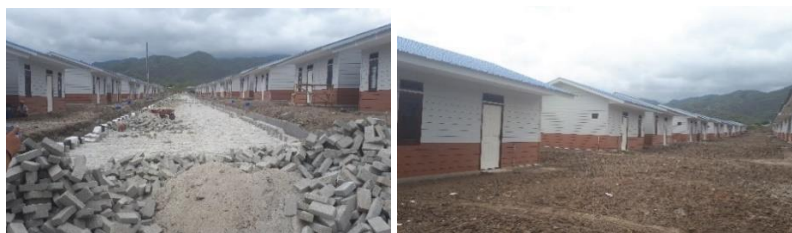
Figure 8. Housing Construction Condition in Palu Source: (Field survey, 2020)
