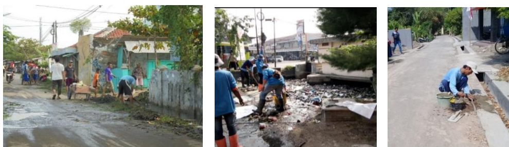
Figure 4. Routine Maintenance by the Community (left), by Local Government (middle) and by Drainage Repair Worker.
